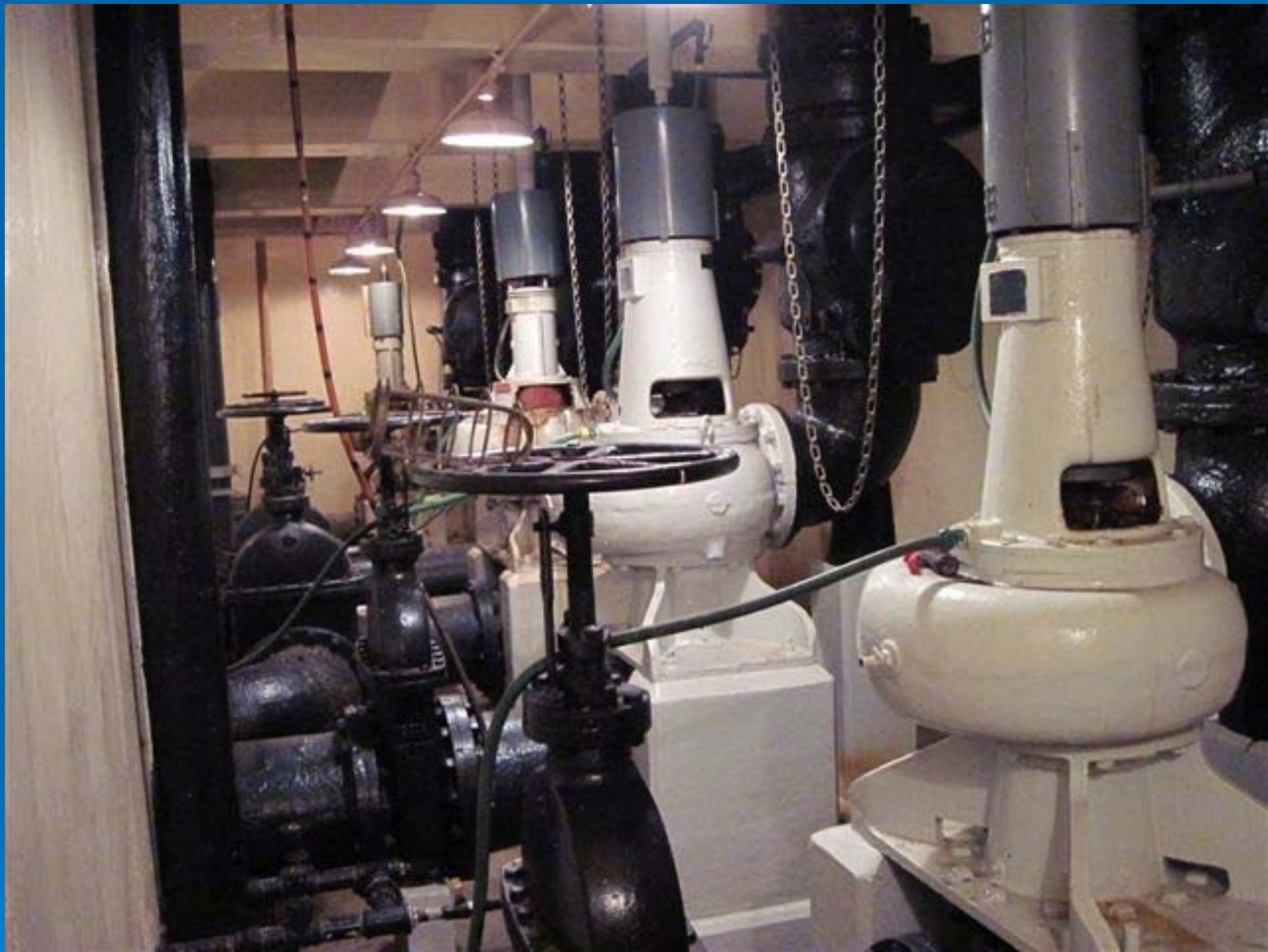
Raw water pumps
