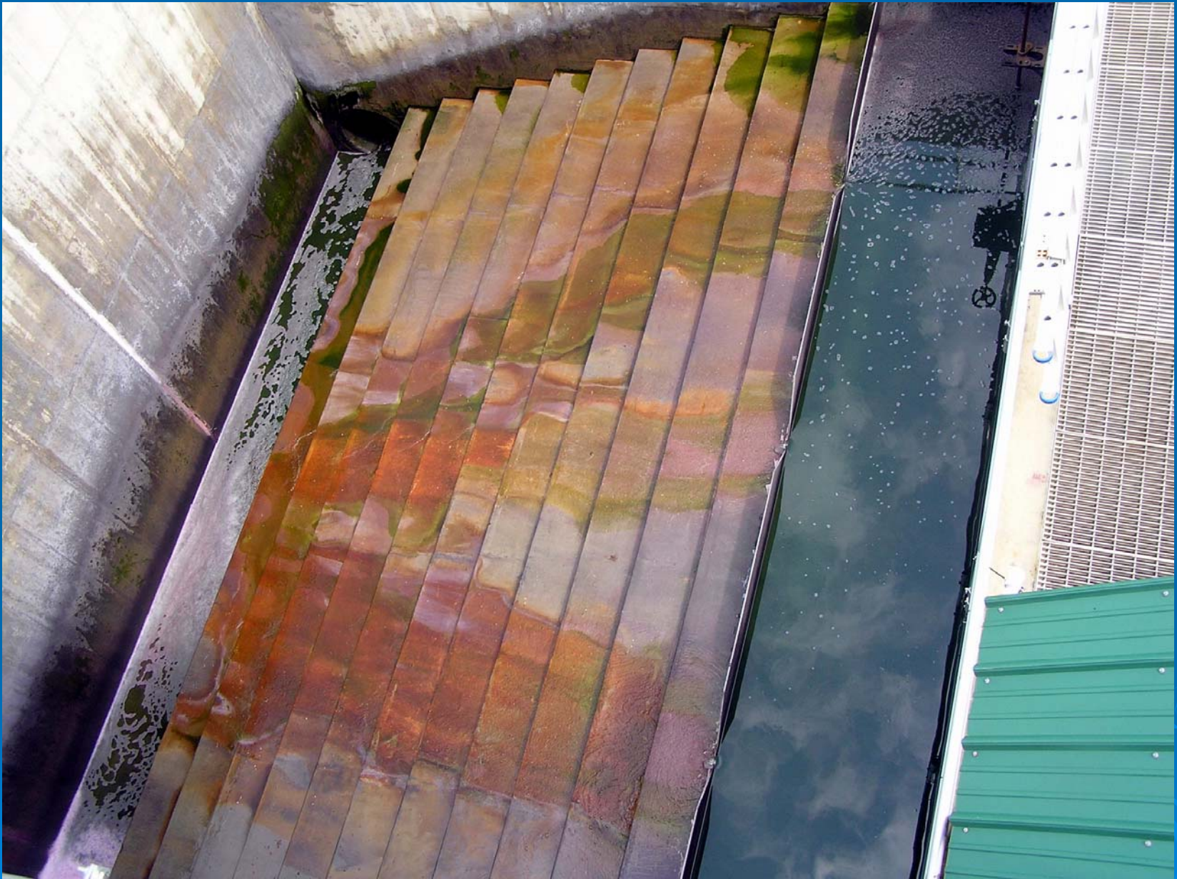
Effluent cascade outfall
