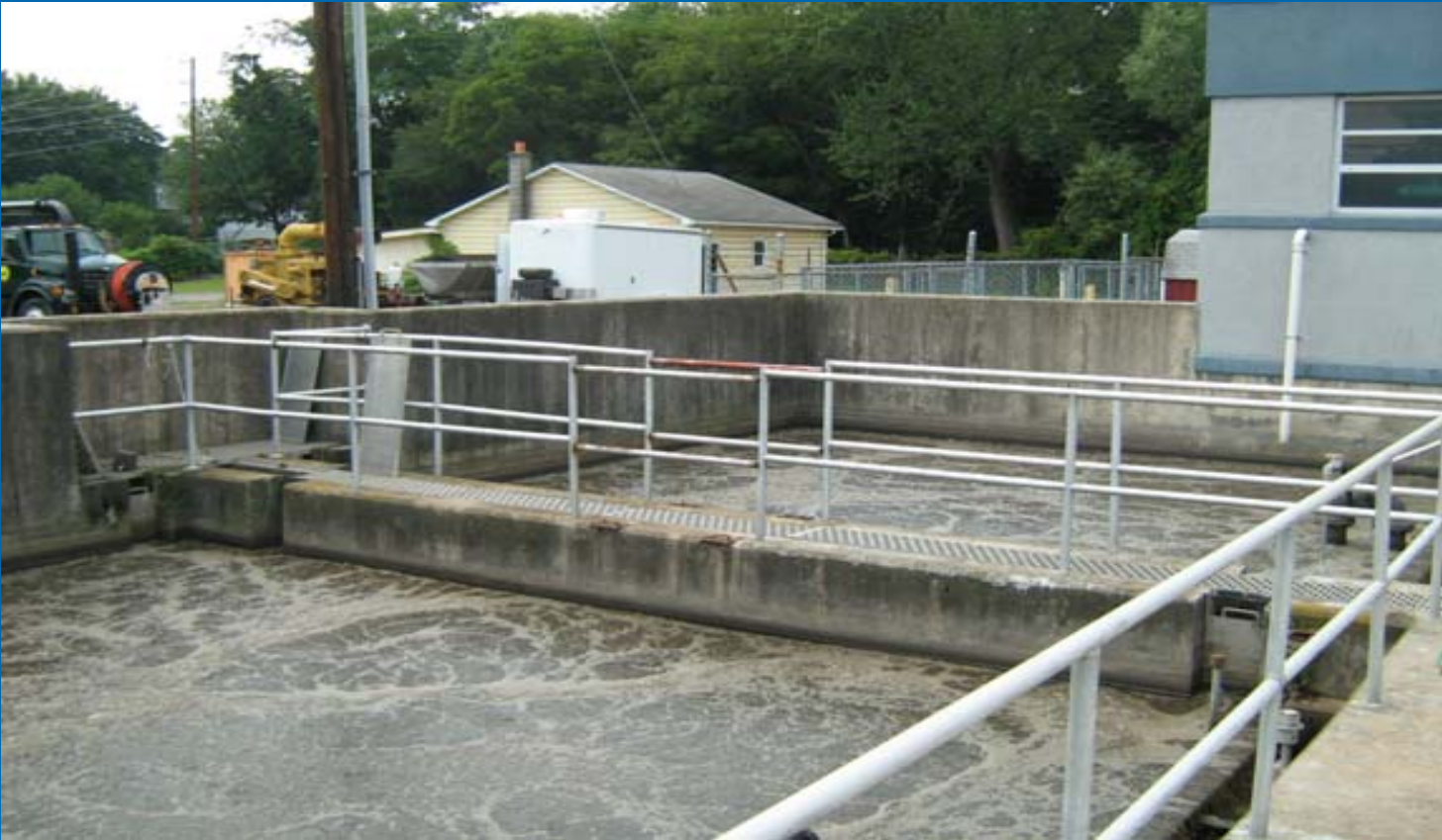
Activated sludge basins
