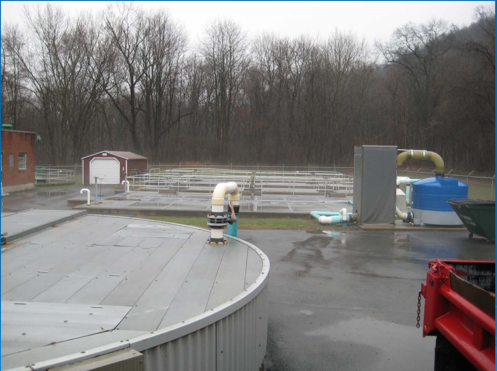
Covered sludge thickener (foreground). Digesters and aeration basins (background).
