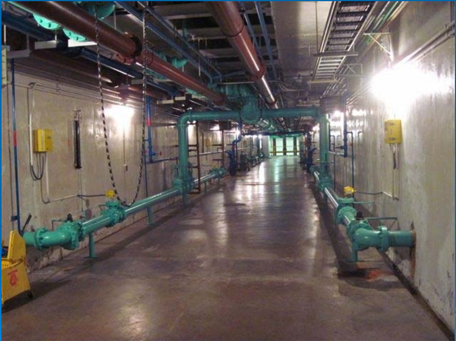
Secondary system pipe gallery
