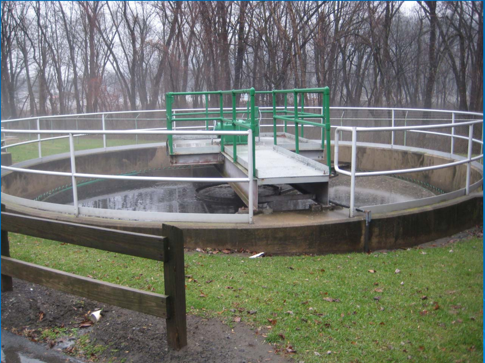
Final clarifier (1 of 2).
