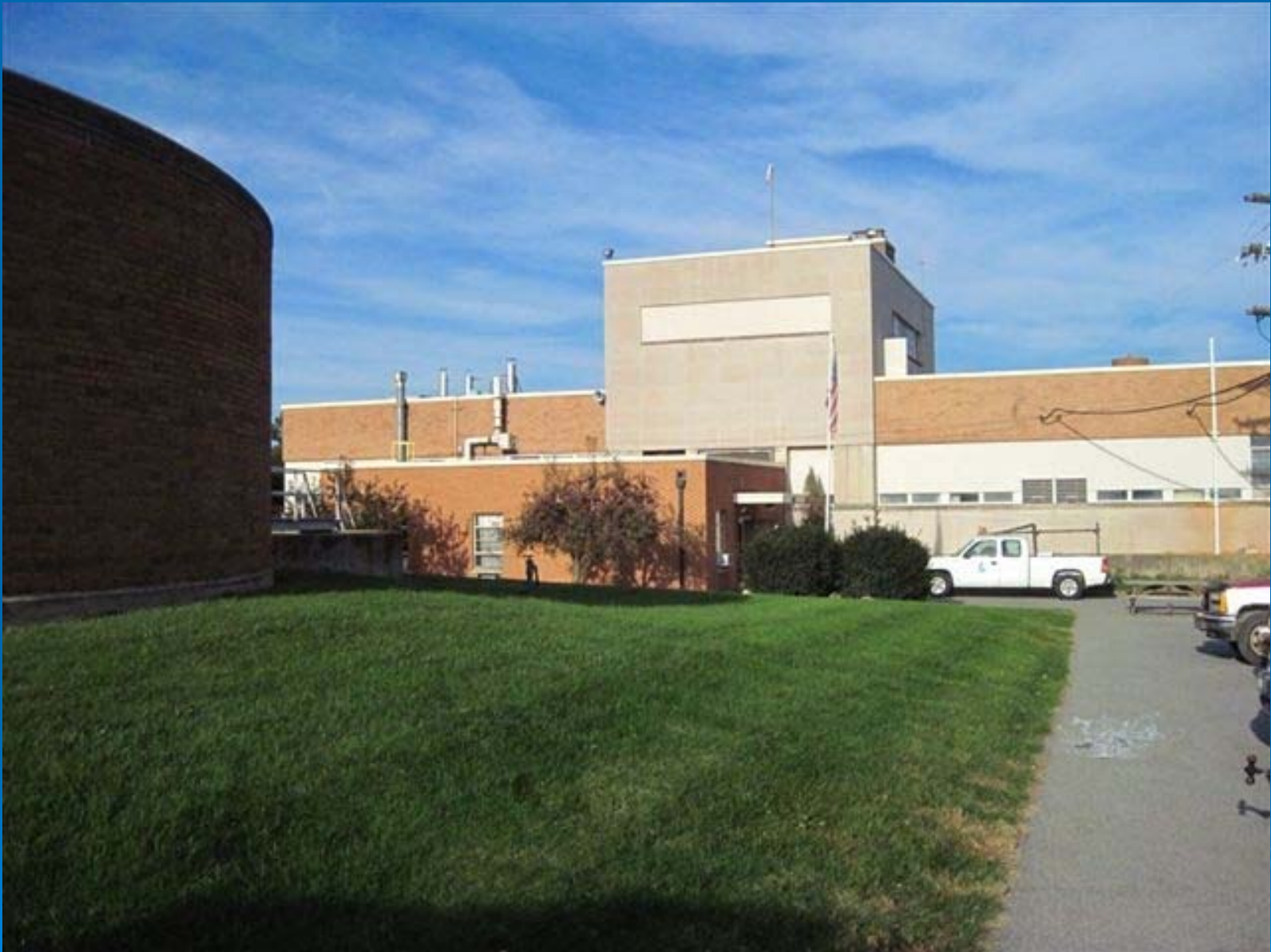
Central Plant Administration Building
