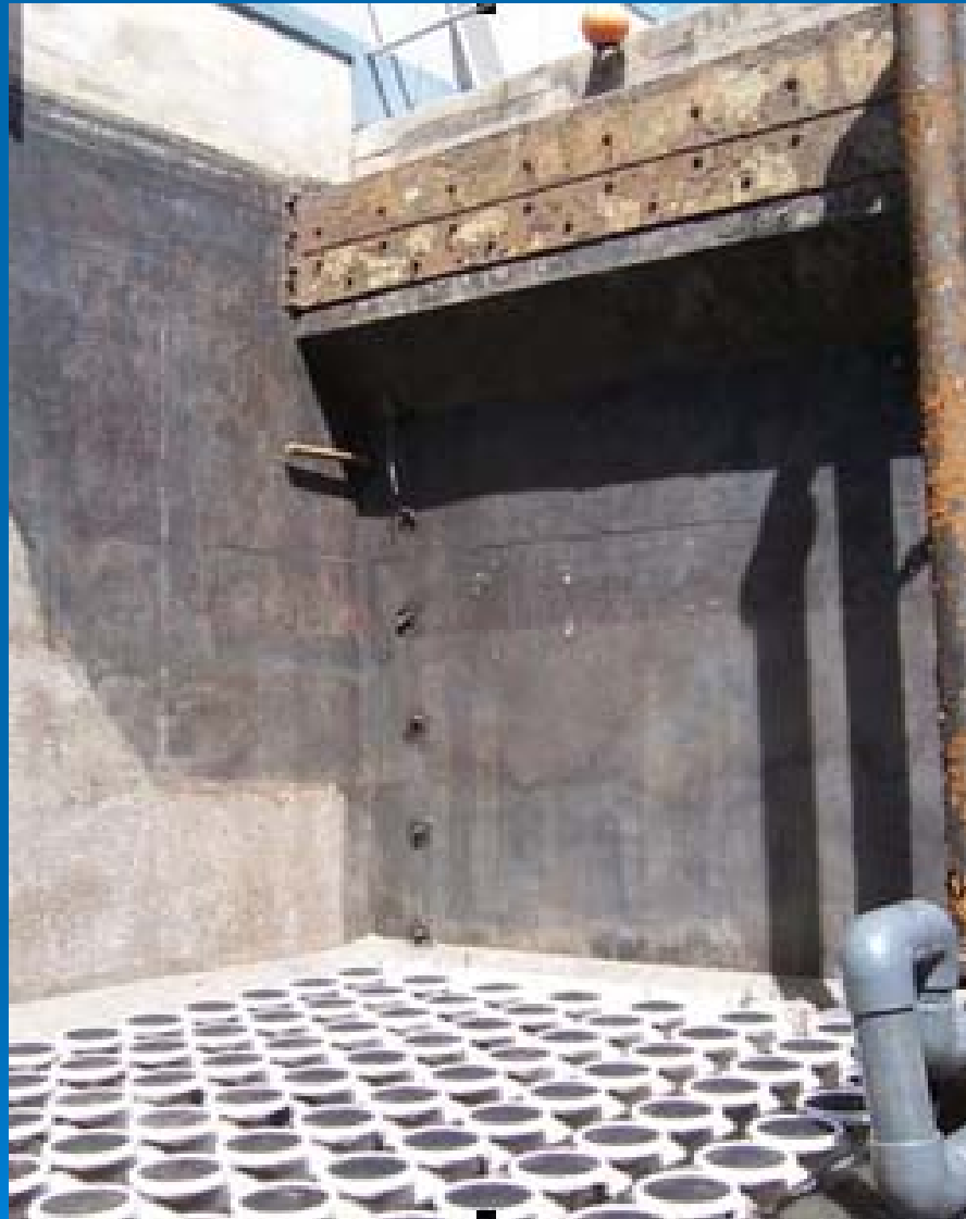
Activated sludge basins—empty, showing fine bubble air diffusers.
