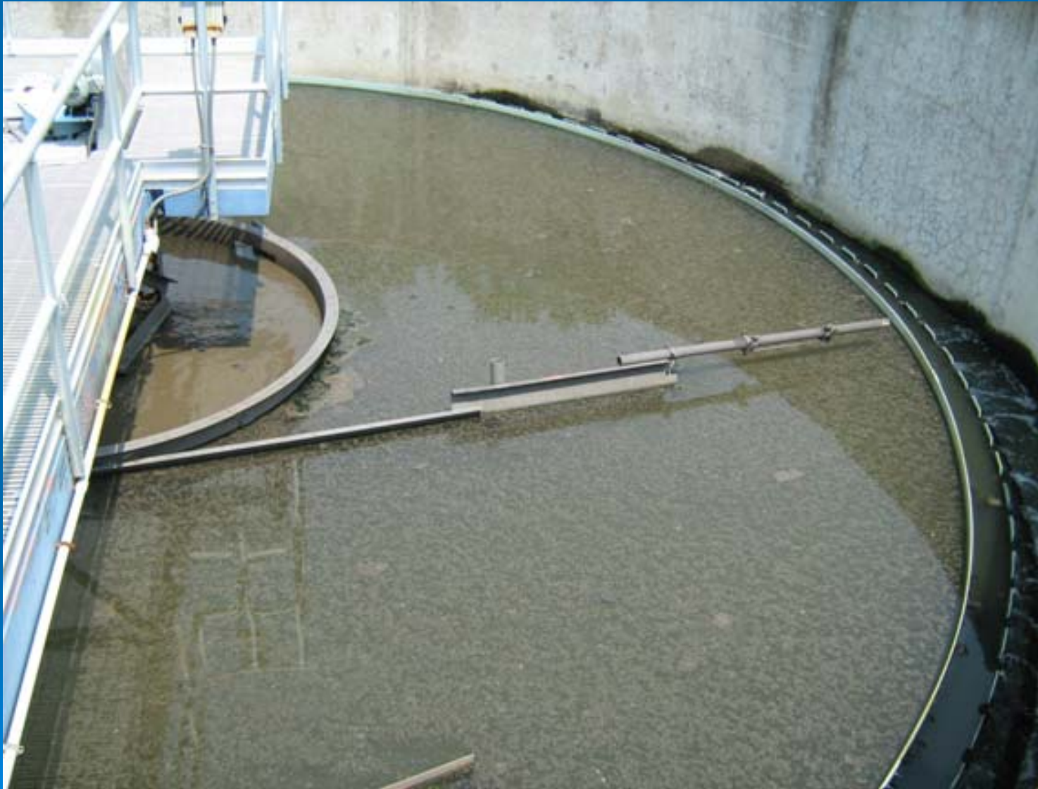
New (1996) final clarifier.
