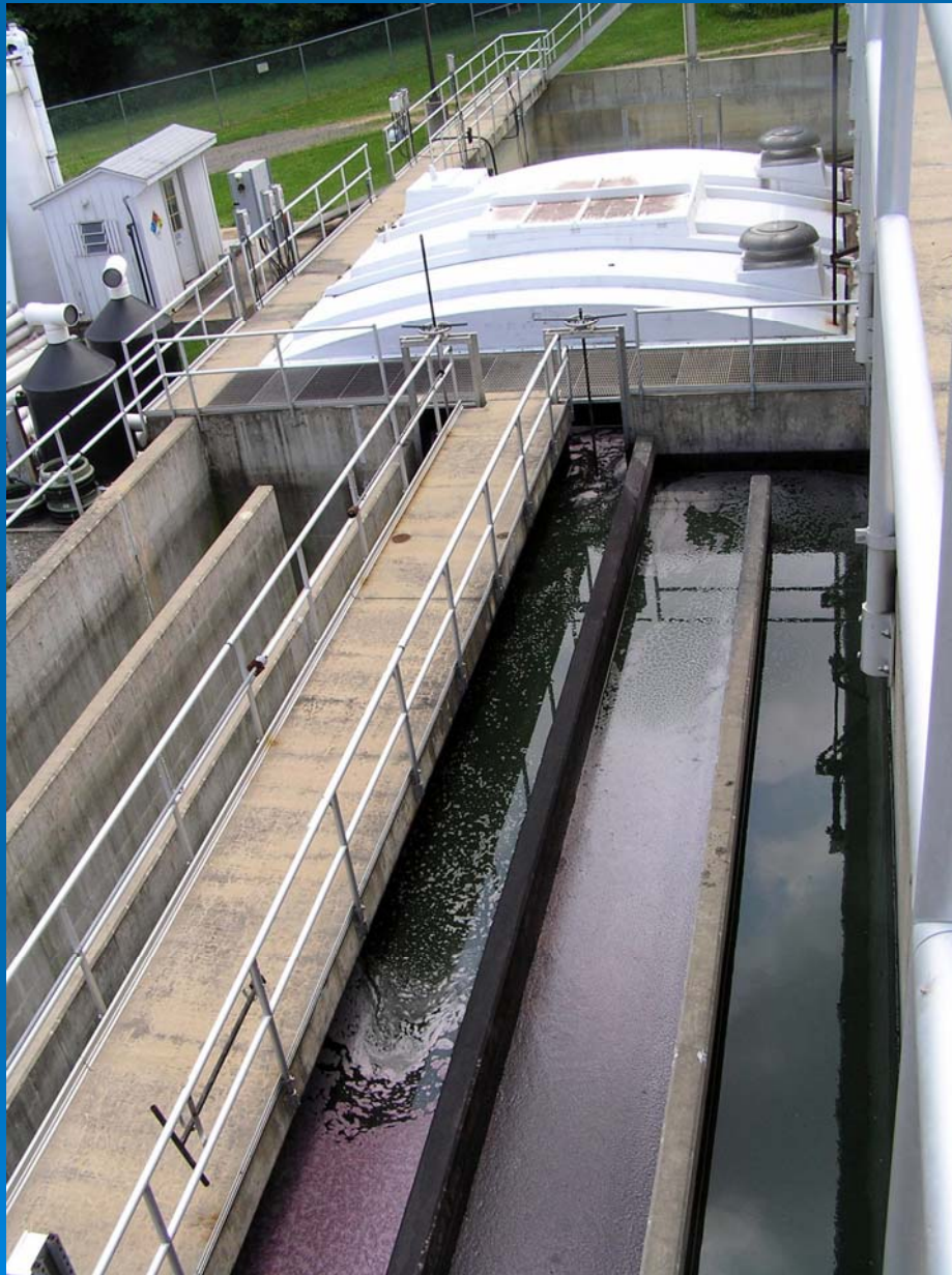
Chlorine contact tank
