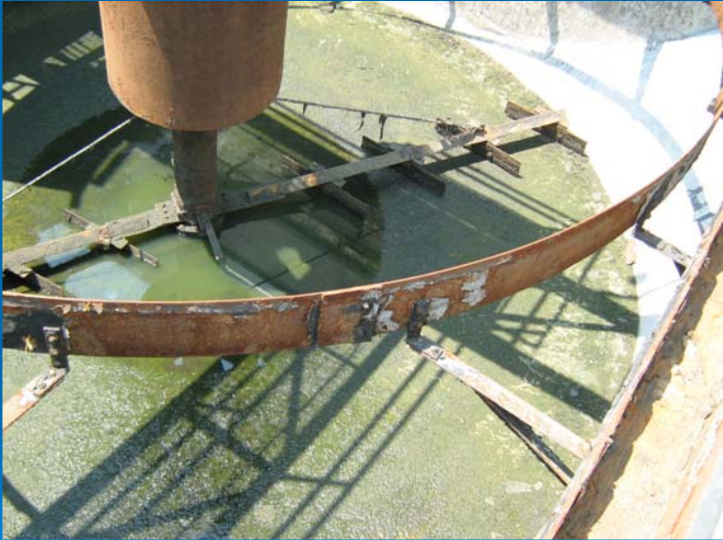
Old (1970s) final clarifier (one of two clarifiers).
