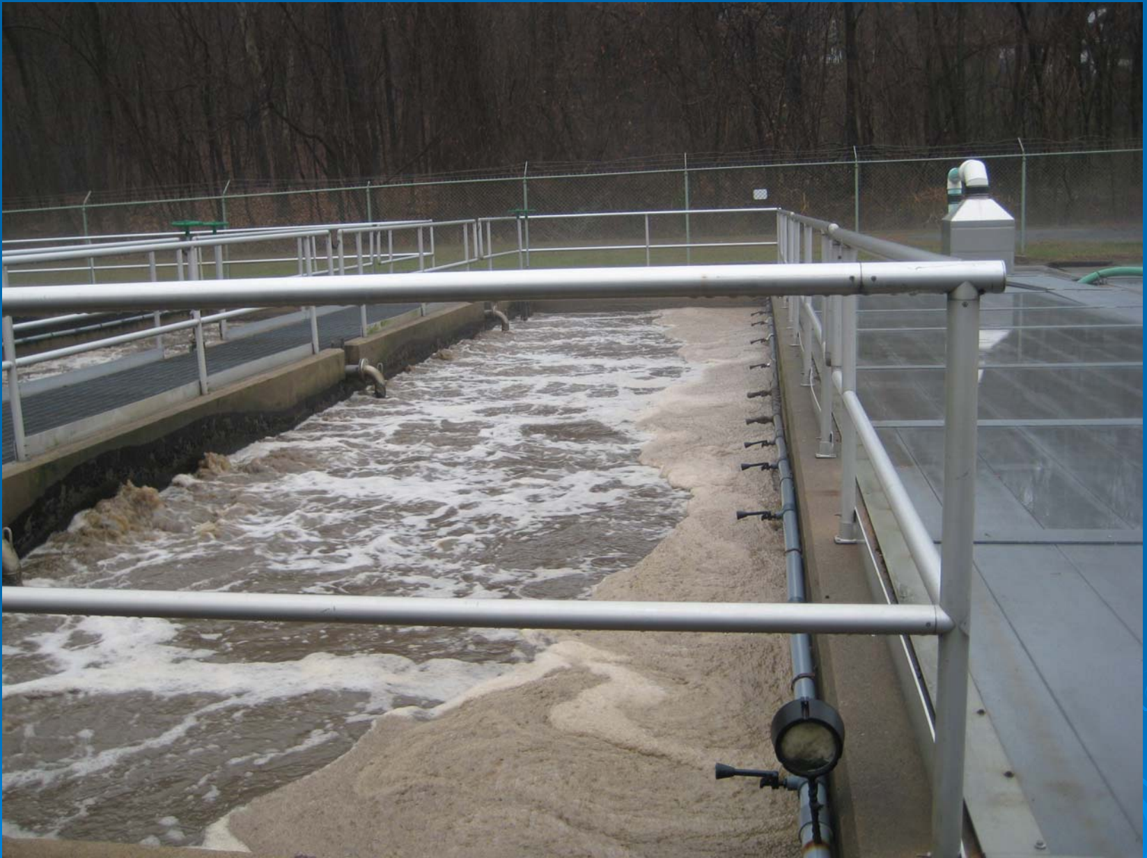
Aeration basin (left) and covered aerobic digester (right).
