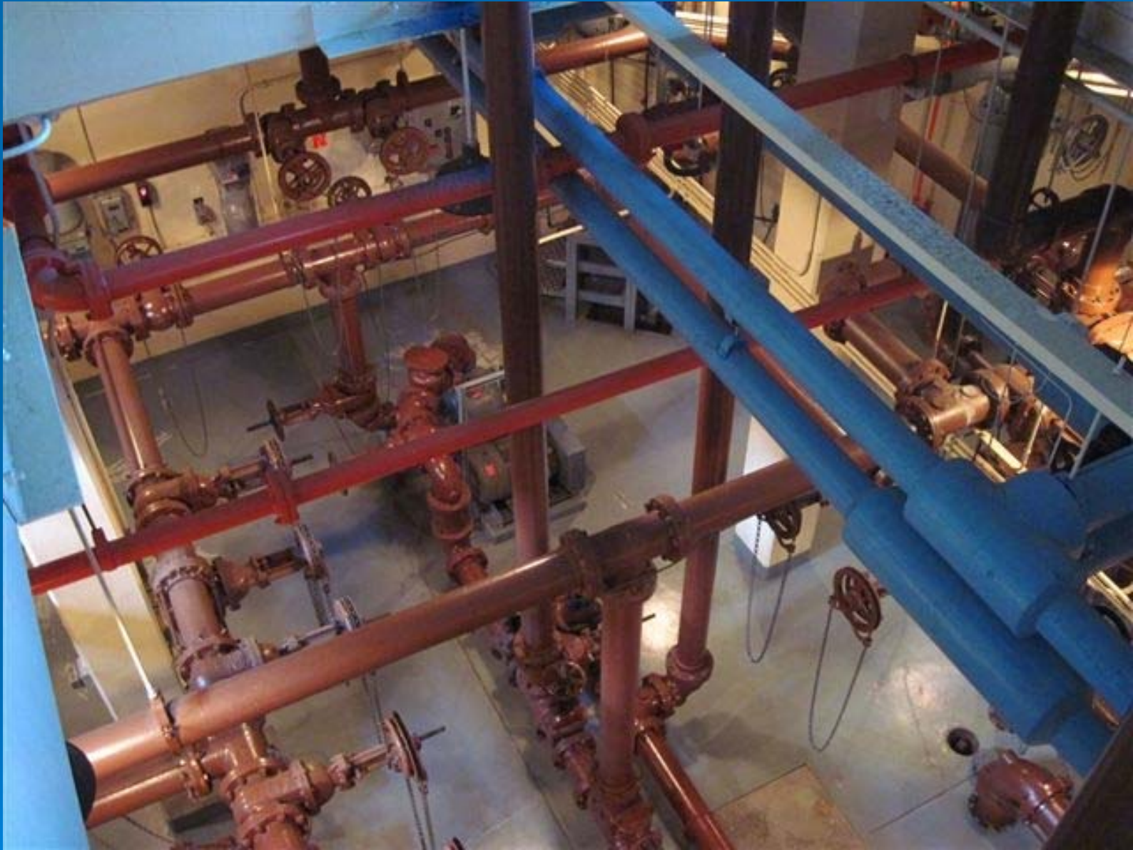
Digester building piping
