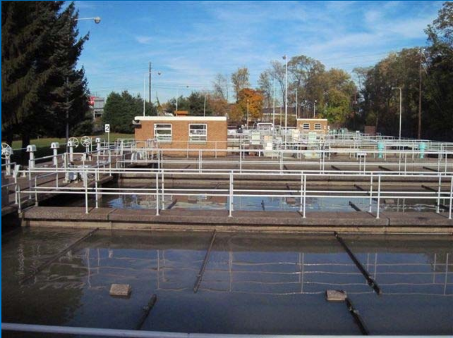
Primary and secondary system tankage
