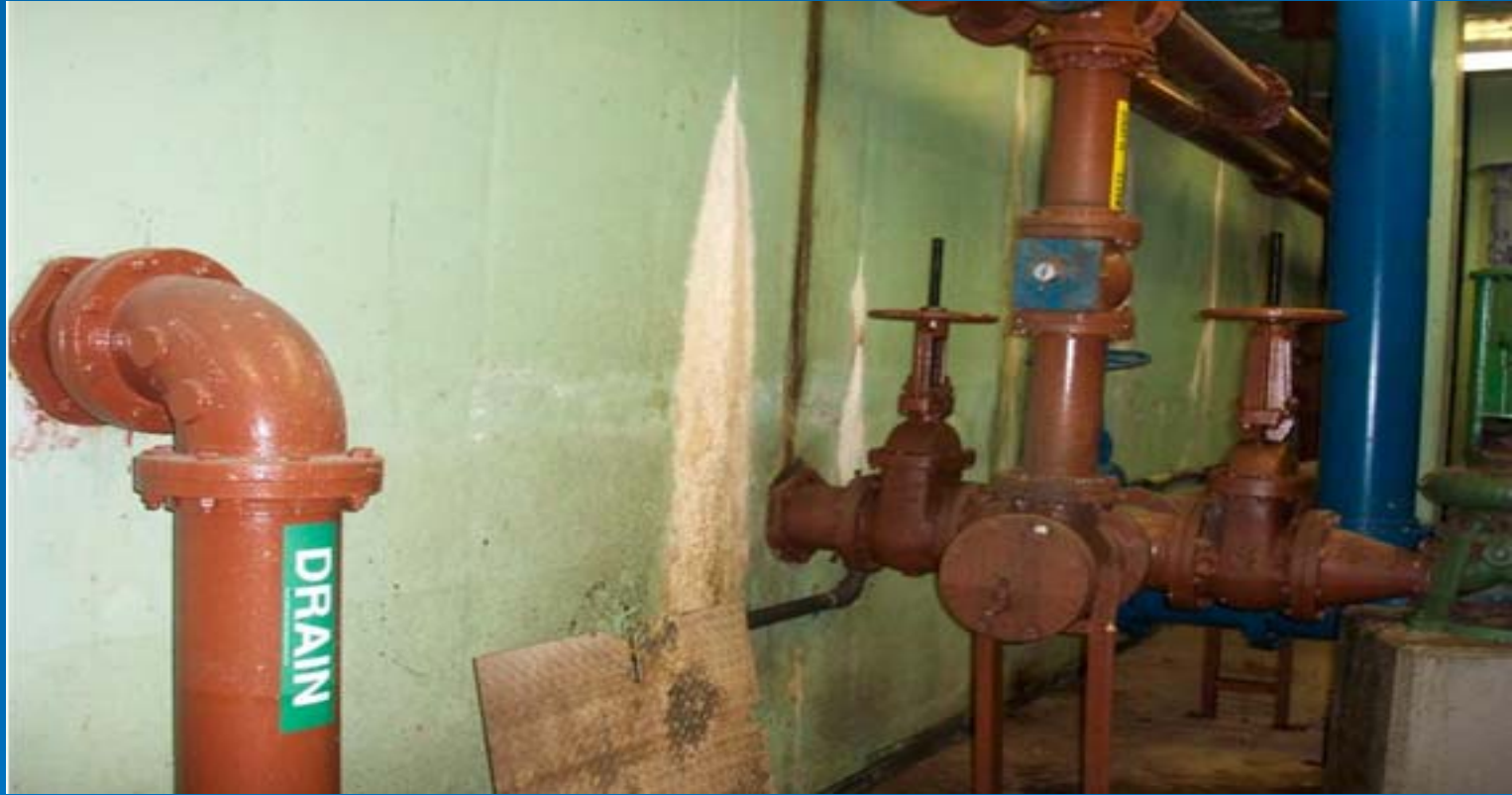
Pipe gallery—evidence of structural damage.
