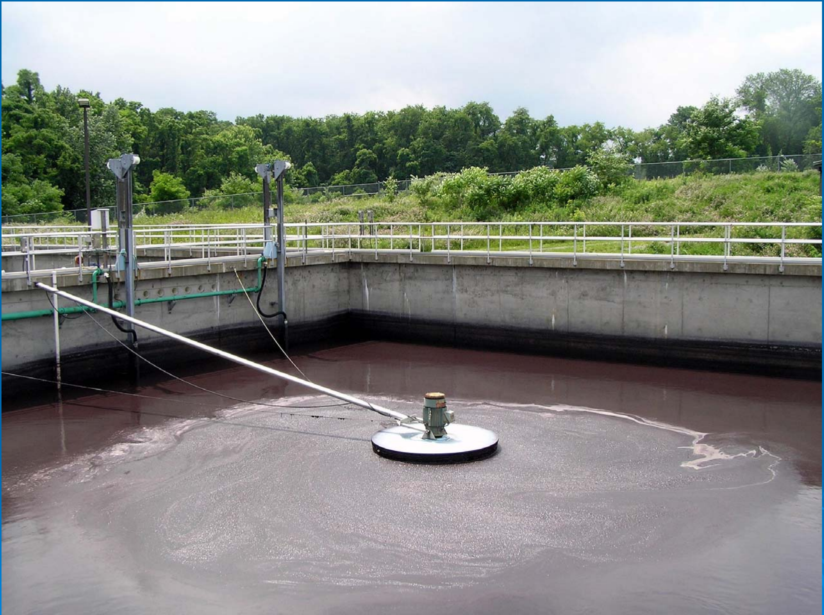
Sequencing Batch Reactor (SBR) tank
